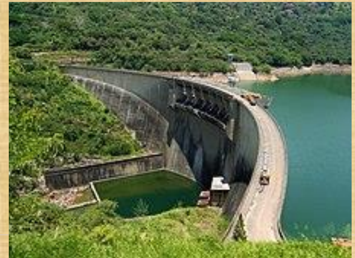
Hydropower plant, Srilanka
