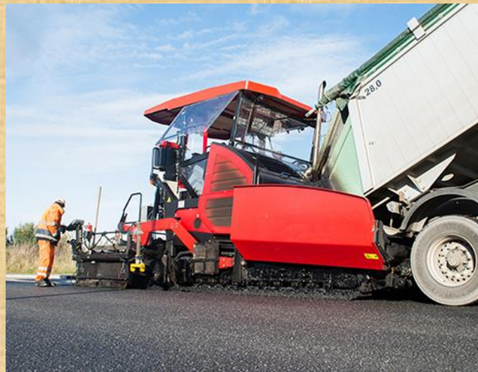
Road construction, Vietnam
