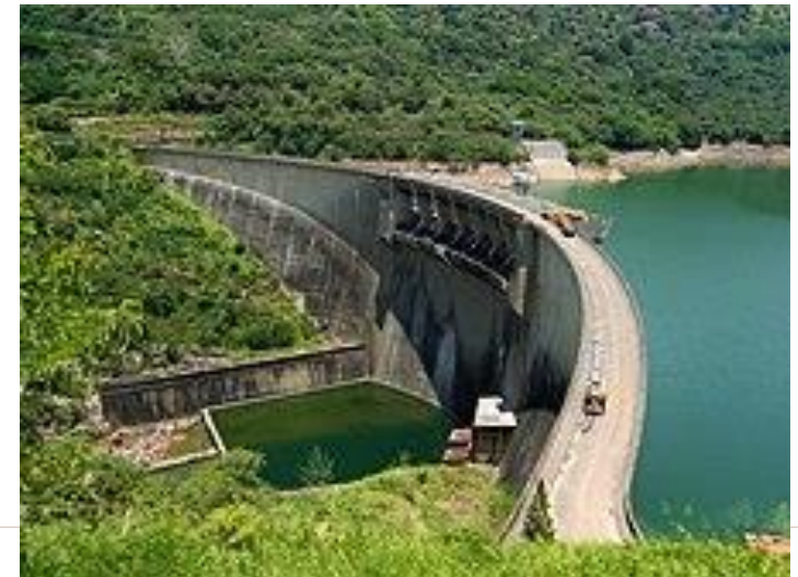
Hydropower plant, Sri Lanka
