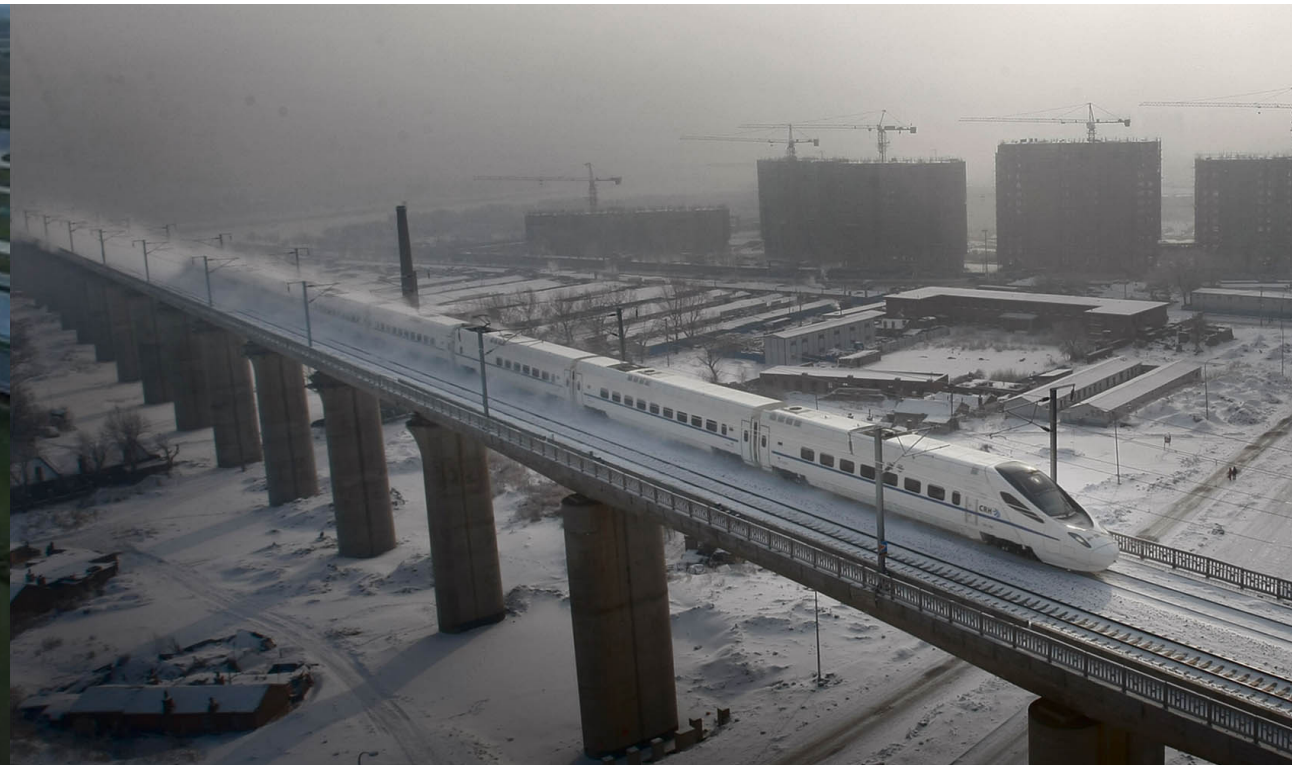
Urbanization along the railway construction
