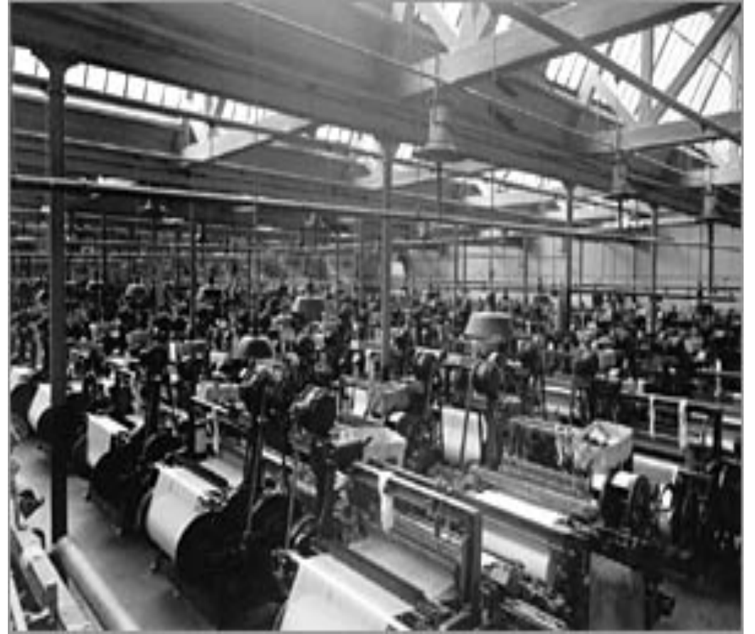
Some of the 1200 power looms at the Plevna factory building, completed in 1877 , at the Finlayson & Co cotton mills in Tampere, Finland.
