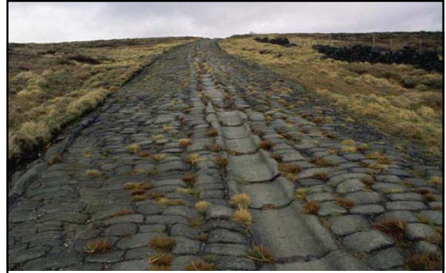
One of the finest examples of a surviving Roman road in Britain, Blackstone Edge, near Manchester, is remarkably well preserved with rain gullies and close-fitting cobbles still intact.
