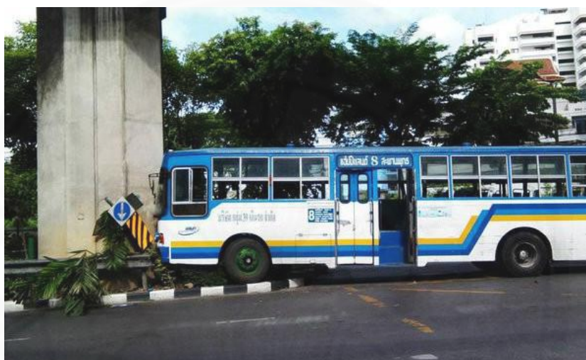
Figure 2.6 Bus Line 8 slammed into concrete pillar
