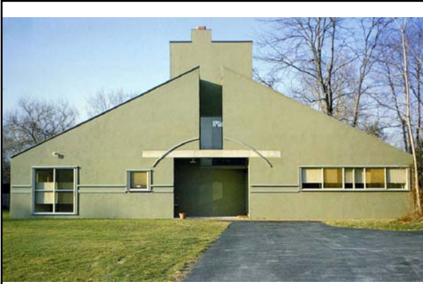
Vanna Venturi house, Robert Venturi, 1962
