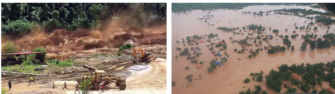
Figure 3 : The damage from the Nam Ao dam collapse in 2017 (left picture) and Xe-Pian Xe Namnoy Dam in 2018 (right picture)
