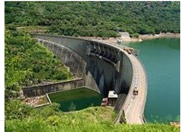
Hydropower plant , Sri Lanka
