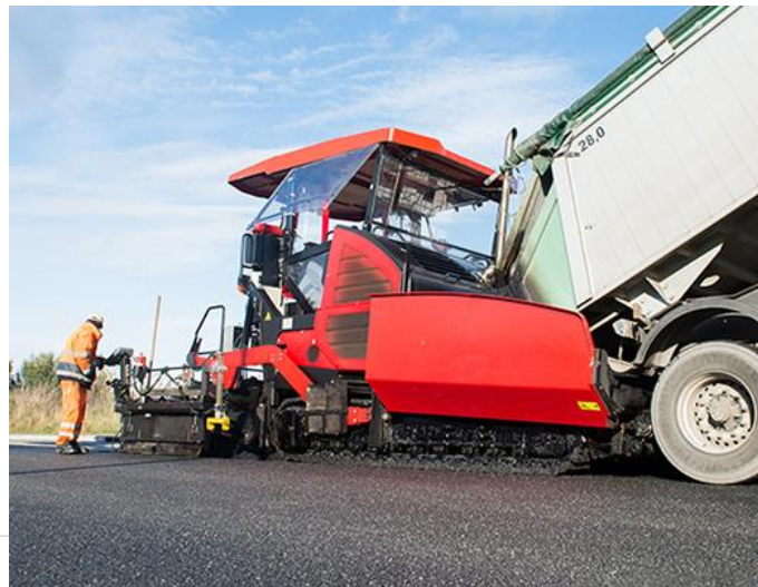
Road construction, Vietnam
